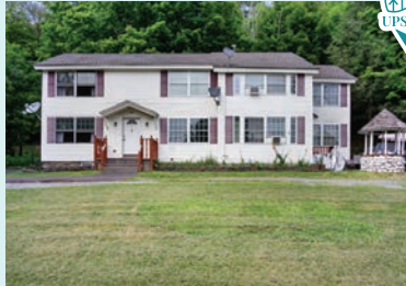
82 High Street Monticello NY 12701
